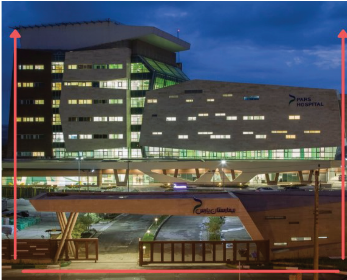
Hospital Pars (Archdaily,2012)
